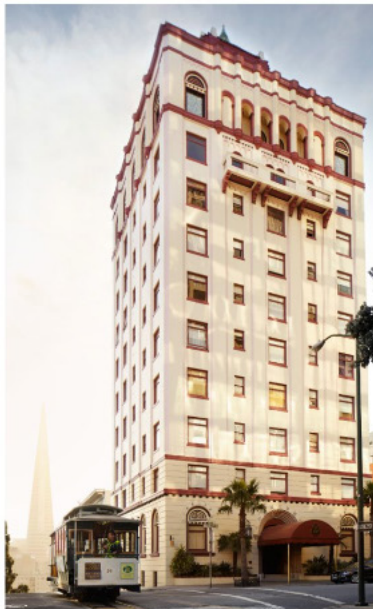
The majestic, 10-story Bently atop San Francisco's Nob Hill was built in the Art-Deco style in 1924. Photo by Michal Venera
